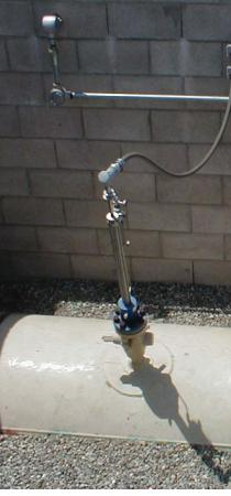
The Elster Instromet CheckSonic Single Path Ultrasonic Flow Meter is one-of-a-kind. With easy to install hot tap, inserted through a 2" or 3" full-port ball valve, retractable transducers, sophisticated digital electronics and the unique bounce path configuration results in a meter ideally suited for certain gas measurement applications. The proven accuracy (better than  $\pm$  1.0%), repeatability and linearity make the CheckSonic one of the world's finest non-custody transfer meters.
