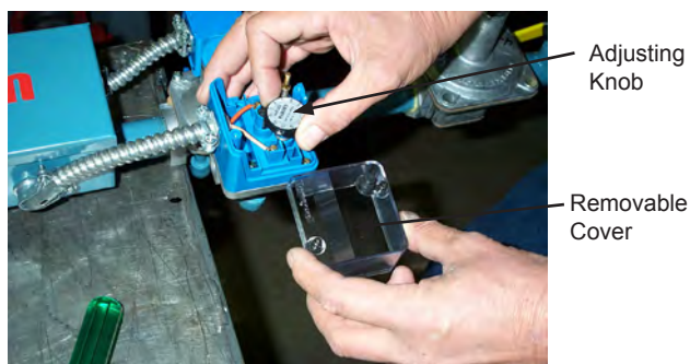
Figure E-8 Gas Pressure Switch Adjustment
