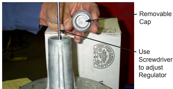
Figure E-7 Main Gas Pressure Regulator Adjustment
