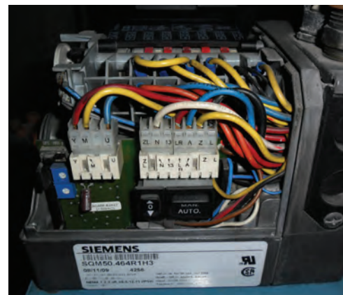
Figure B-18 Siemens Mod Motor Adjustments
