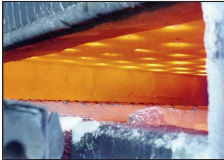
Roof Mounted WHG Burners on Aluminum Melting Furnace
